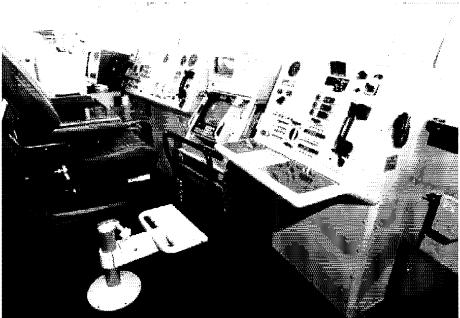
Figure 18.5. Bridge of a Type 23 frigate (Reproduced with permission from MoD/BAE SYSTEMS Marine).
